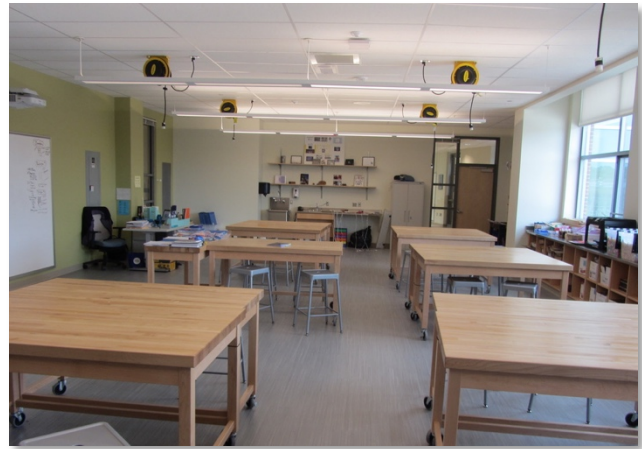
Ceiling bar (left) and electrical drops (right).
