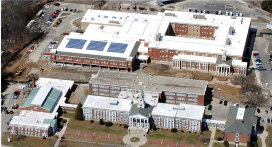
Aerial view of the new Norwood High School, the MSBA's first Model School, situated behind the existing Norwood High School.
