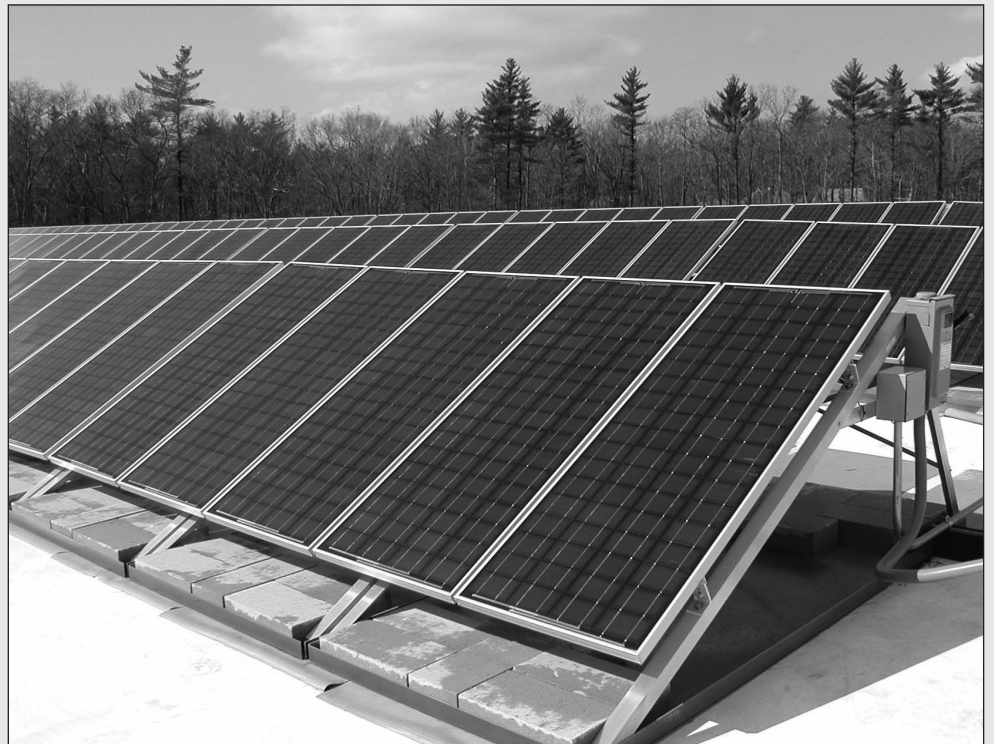
Top photo, view of the library at Whitman-Hanson Regional High School. Above, view of the exterior of the school. At right, a 51-kW solar electric system installed on the school's roof supplies approximately five percent of the building's annual energy use.
