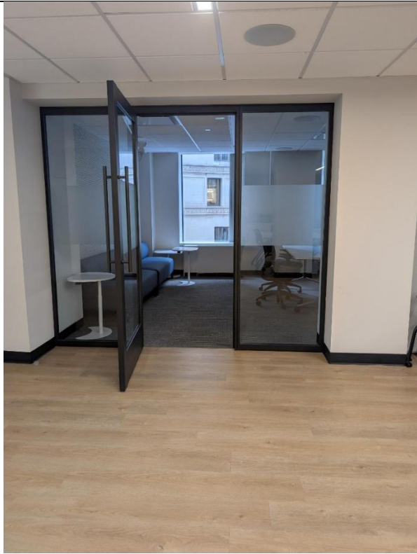
Example: Glass partition installation, Board Room
