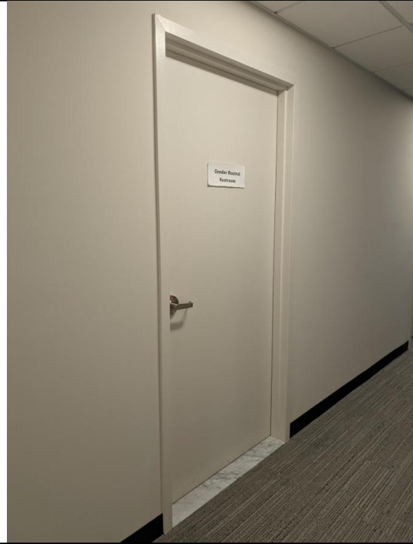
Example: Identification of room use at door according to ADA requirements, drywall surface. Gender Neutral Bathroom
