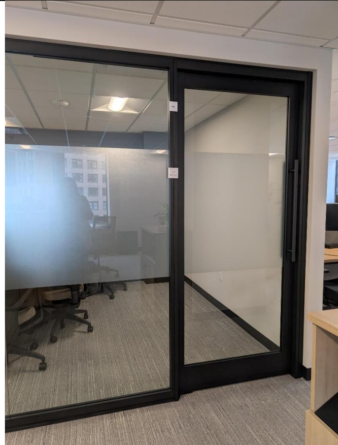
Example: Glass partition installation, sliding door closed
